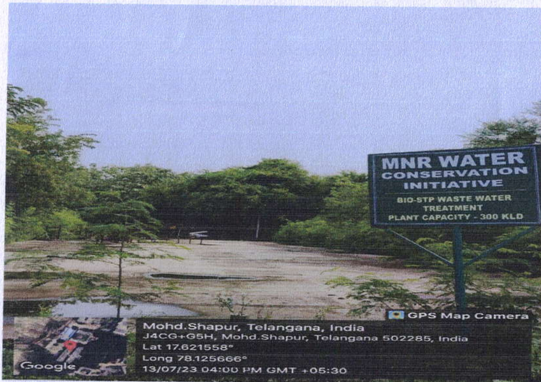
MNR WATER CONSERVATIVE INITIATIVE-BIO STP WASTE WATER TREATMENT PLANT CAPACITY-300KLD
